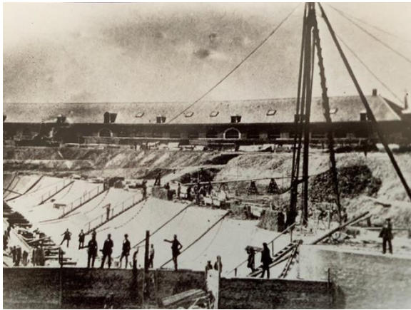
Bouwput Dok II
